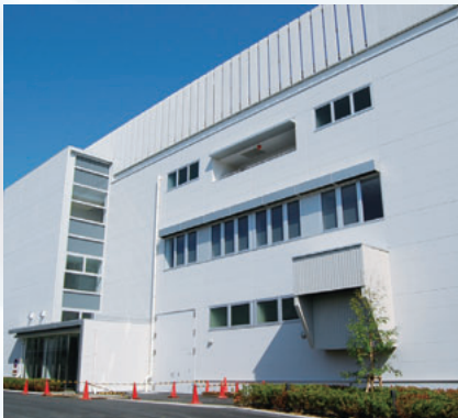
The newly constructed Tsubaki Group Auto Engineering Lab
