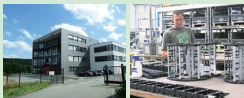
KS headquarters building and cableveyor production site
