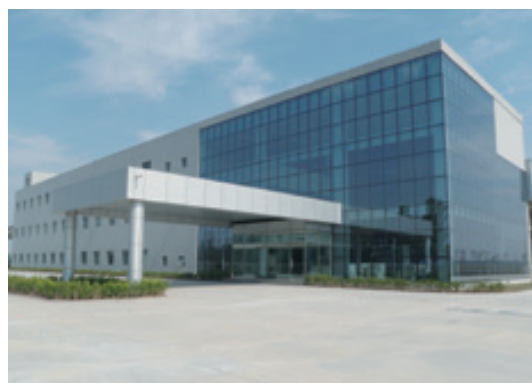
Second factory of Tsubakimoto Chain (Tianjin) Co., Ltd., where operations commenced in August 2015 (China)
