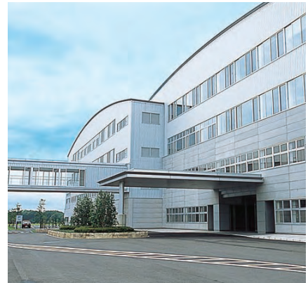
Technical center at the Kyotanabe plant
