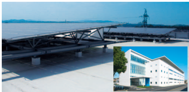
Solar panels at new assembly factory building in the Saitama Plant
