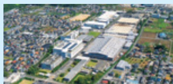
Photograph is of current Saitama Plant
